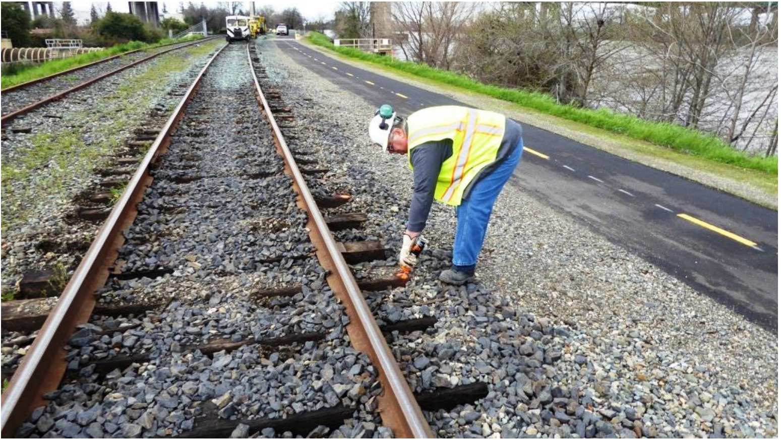
Chris marks bad ties for removal
