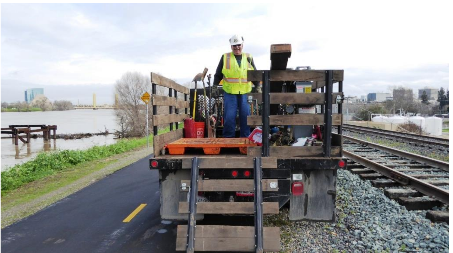
Harry disseminates track-jacks and tools from the bed of the truck
