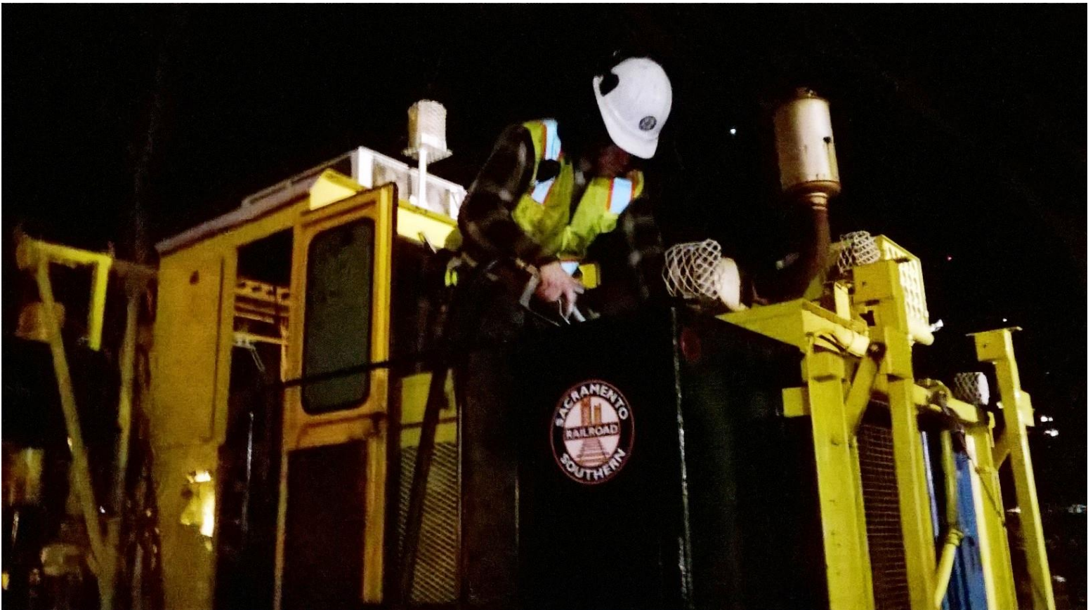
Matt fills the tamper's green diesel tank
