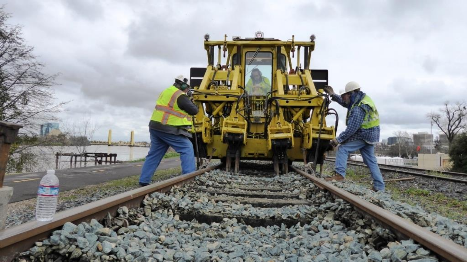
Chris and Mike M. remove the jacks as Alan in the tamper tamps the track to the new level (is a bottle of water on the head of the rail a violation of any provision of Part 214?)
