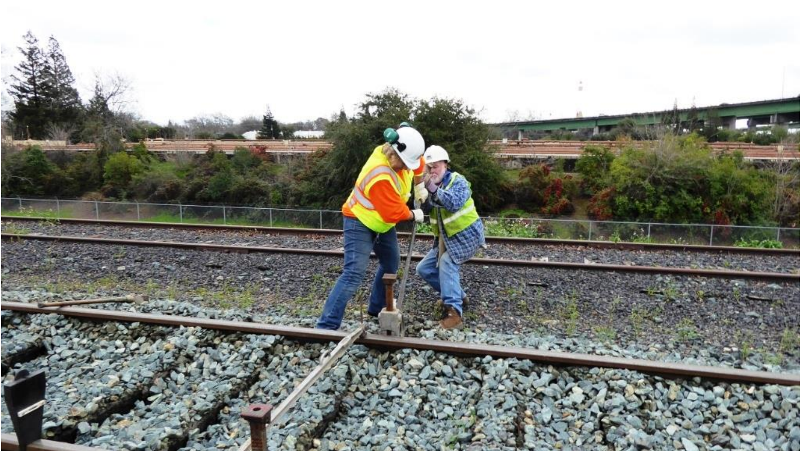
Bev and Mike M. combine efforts to bring the east rail level with the west
