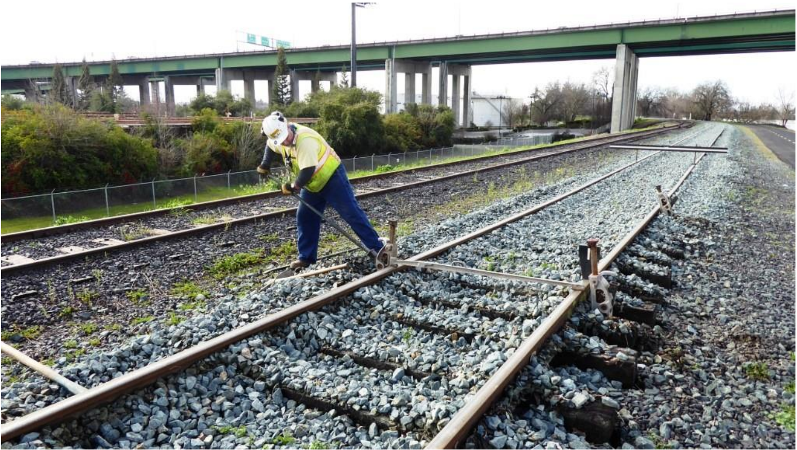
Mike F. jacks-up the east rail making it level with the west
