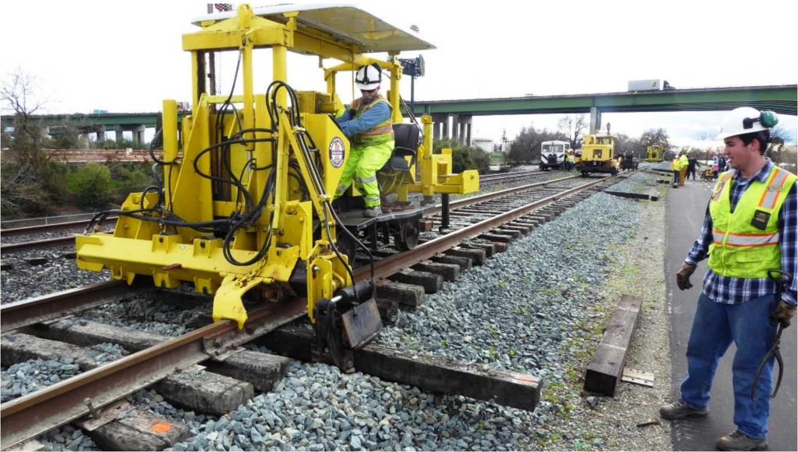
Joe on the 125 pulls another dead tie out from under the rails as Weston stands ready to grab it and get it out of the way
