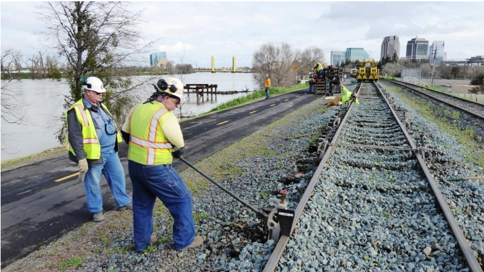
Alan, behind the "hound" signals to Mike F., at the "hare", to crank on that jack
