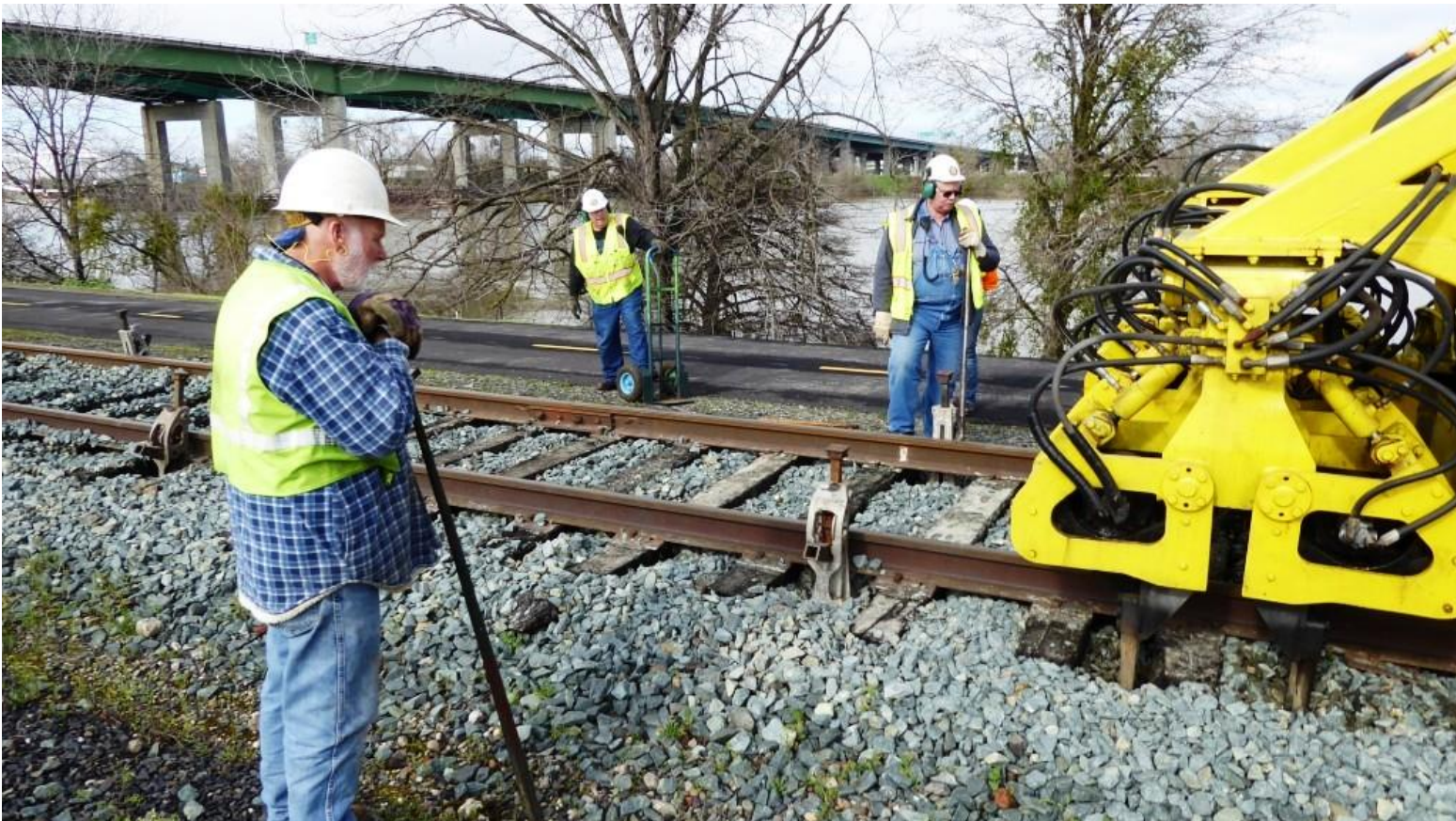
As the tamper approaches, Mike M. and Chris get ready to pull the jacks as Harry waits to transport them further down the line
