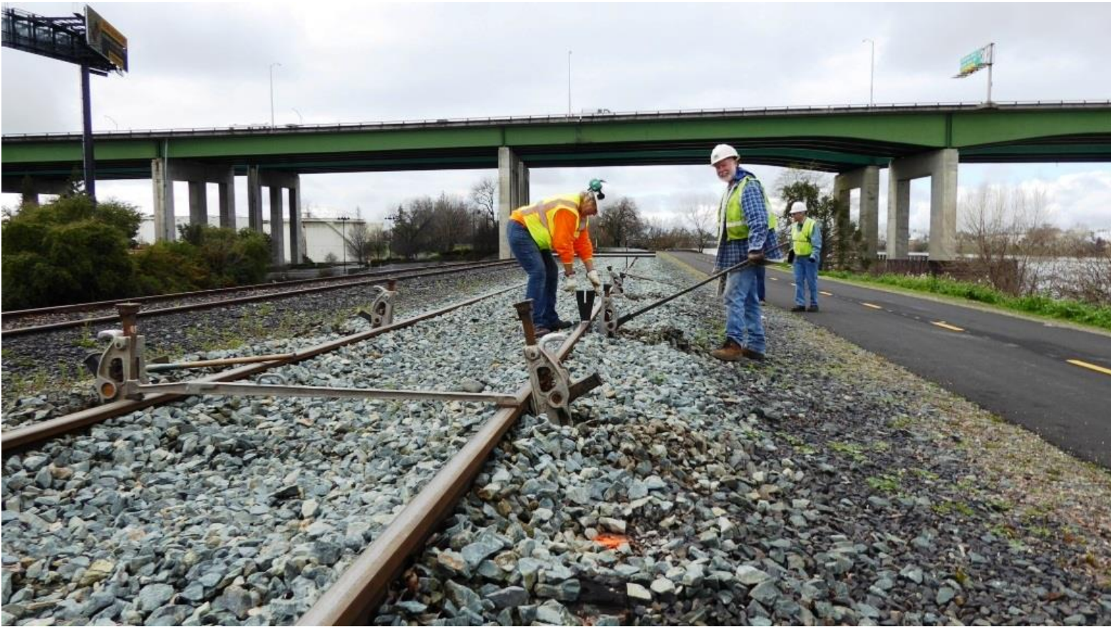
Bev sets up the "hare" at the next jack which Mike M. is ready to raise
