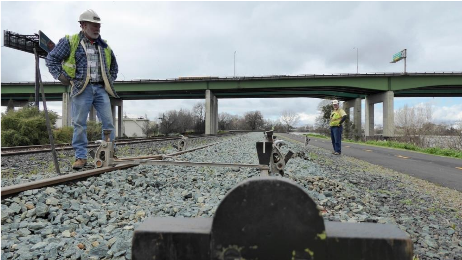
This is the view from the “hound” to the “hare” and on to the spot-board. From the vantage point of the peephole in the “hound”, the vertical white line on the “hare” must reach the horizontal white line on the spot-board as the track is jacked-up
