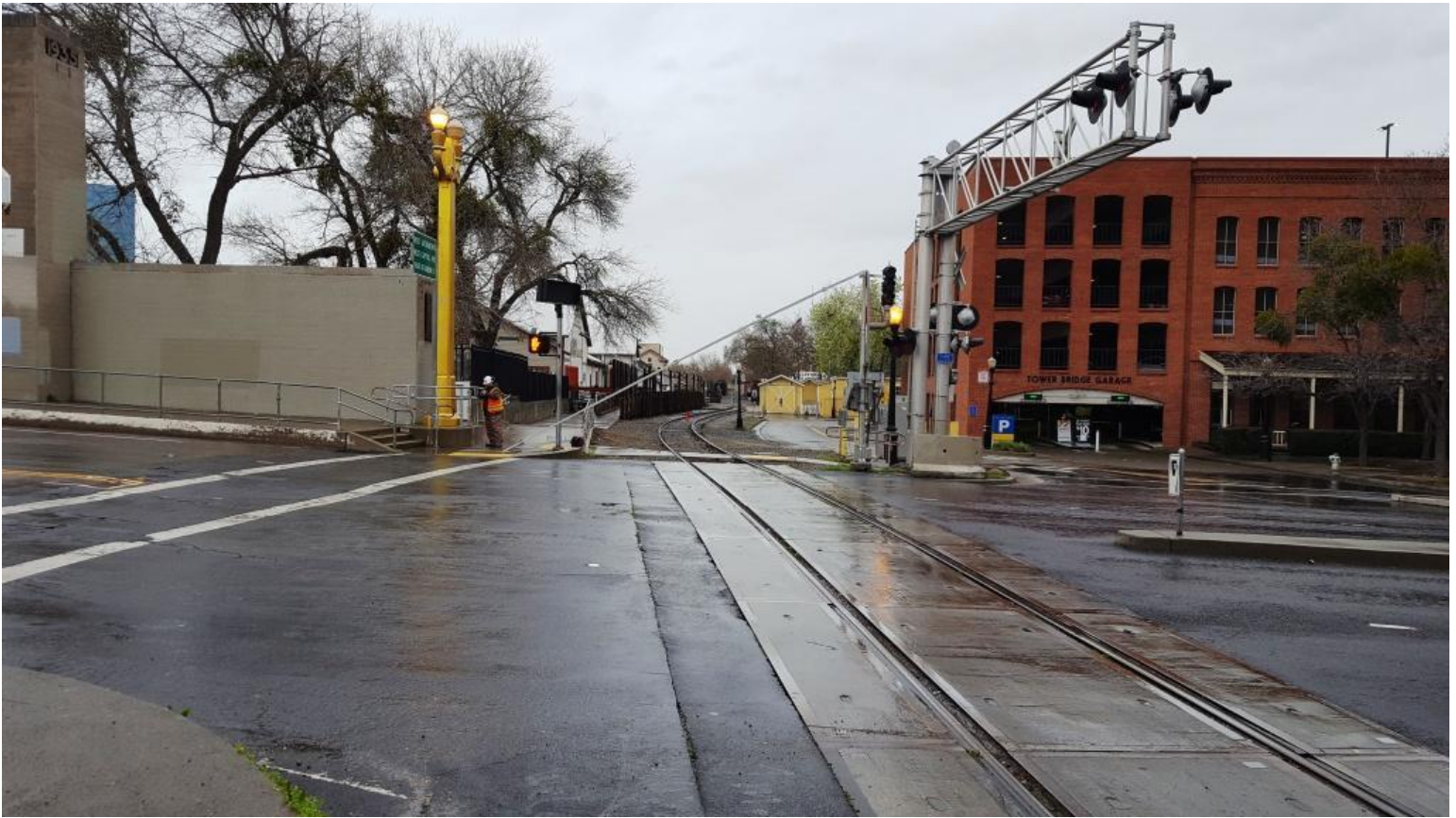
Crossing gate collapse at Capitol Mall
