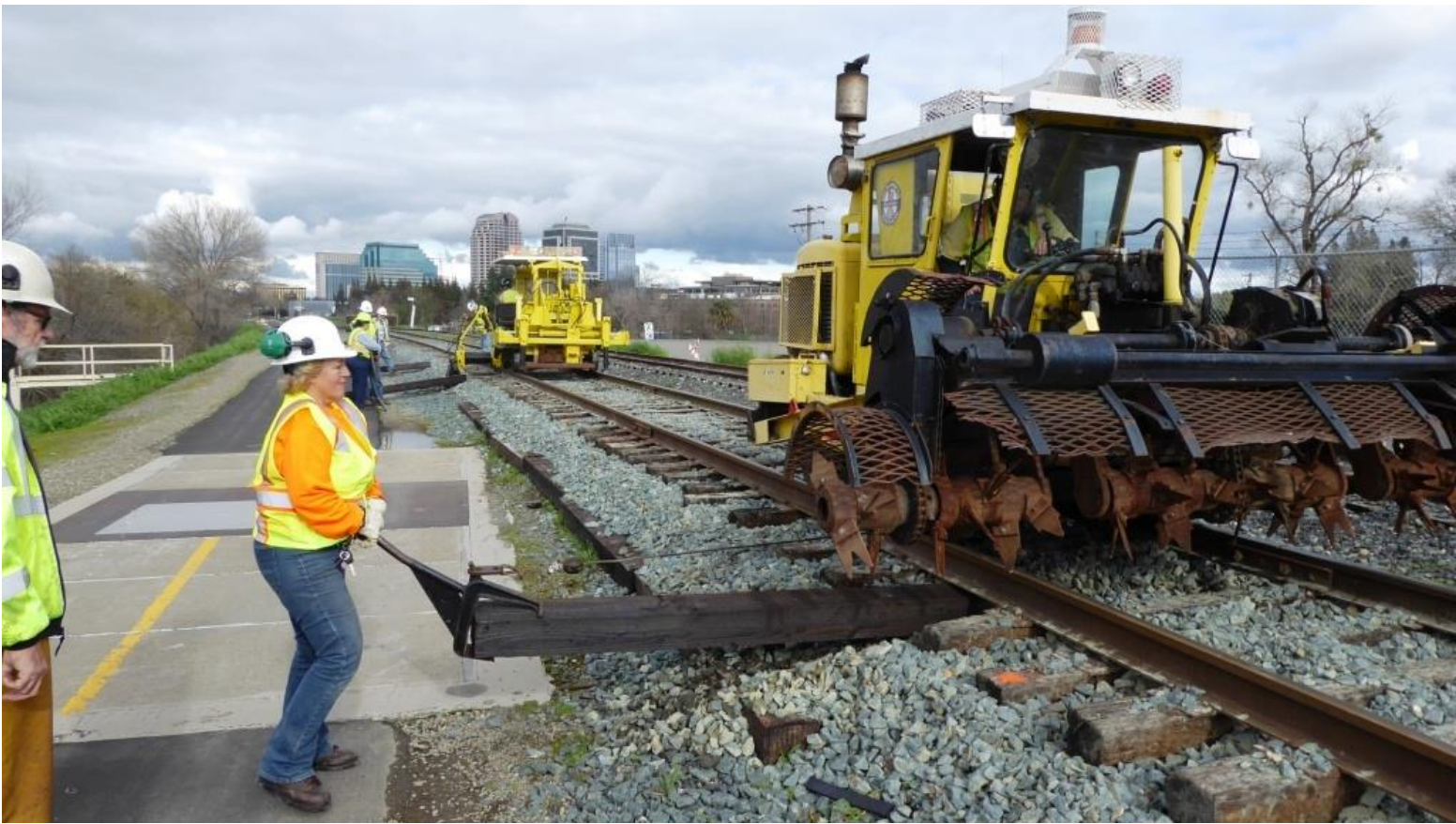
Bev guides a new tie under the rails which Mike F. in the scarifier-inserter pulls in
