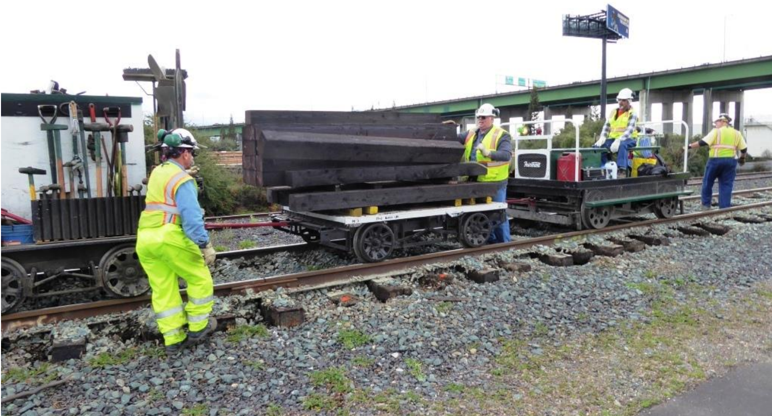
In the afternoon, Joe and Chris distribute new ties to replace those being pulled
