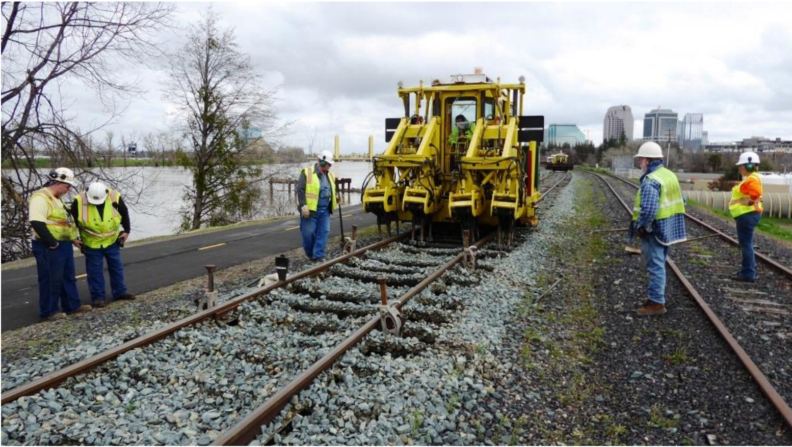
The Team builds a run-off to lessen the severity of the level change
